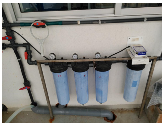
Figure 30 Cartridge filter battery (25 \mu\text{m} , 5 \mu\text{m} and 1 \mu\text{m} ) for FTS continuous circuit seawater filtration. The UV sterilization unit is shown on the right side of the image
