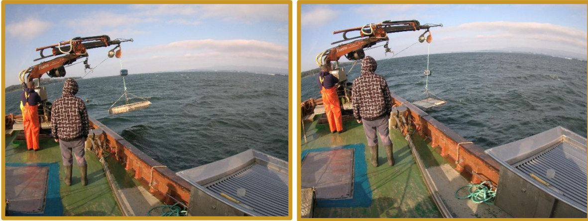
Figure 4. A frame structure with six boxes in the process of submersion in Lombos do Ulla.
